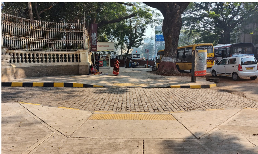
Ramp with drop kerbs and tactile paving for universal accessibility
