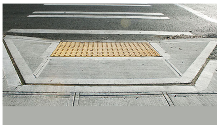
Ramp with drop kerbs and tactile paving for universal accessibility
