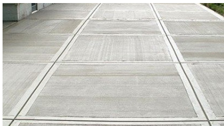
In-situ concrete panels for footpath
