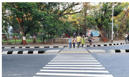
Refuge island for pedestrian crossing
