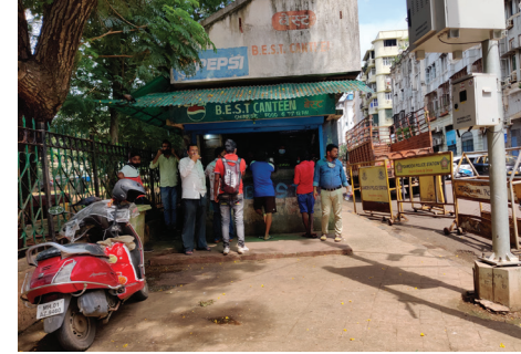
Existing structures on footpath - BEST canteen
