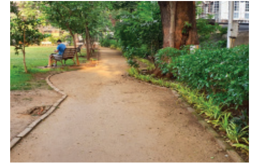
Creation of internal permeable mud macadam pathway
