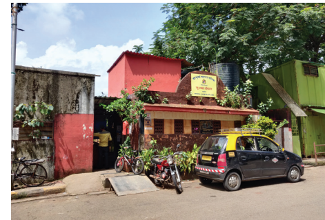
Existing structures on footpath - Sulabh Shauchalay
