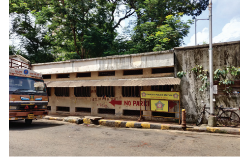
Existing structures on footpath – BEST canteen and shelter
