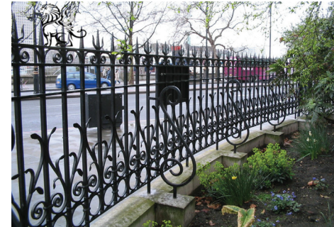
Restoration and reinstallation of gates and peripheral fencing
